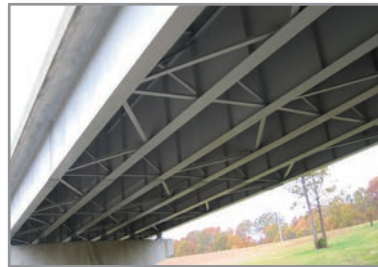
Rust Grip® on Vicksburg Bridge
