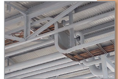
Rust Grip® applied to BP Fuel Terminal, Birkenhead, South Australia
