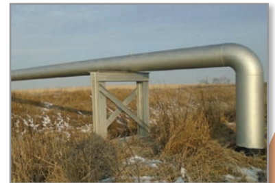
Pipelines in difficult environments
