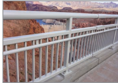
Hoover Dam project with Rust Grip®, Super Therm® and Enamo Grip®
